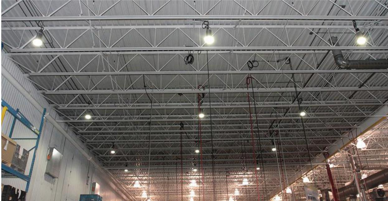
Figure 1 Magna AutoSystems 122watt LED HiBays
